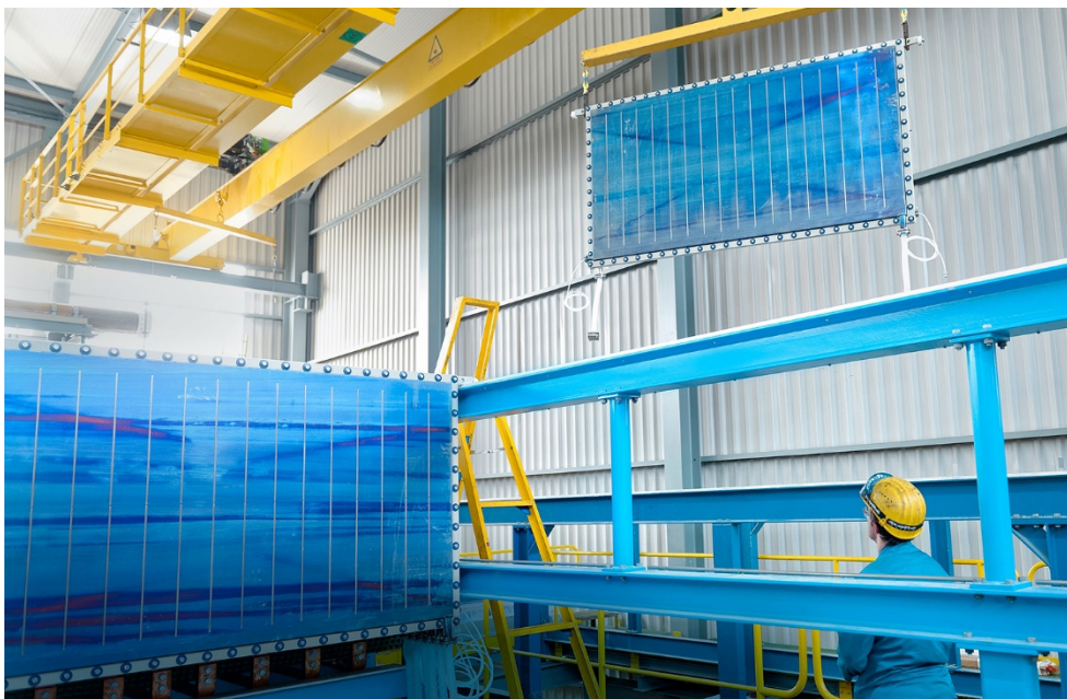
Assembling electrolysis cells
